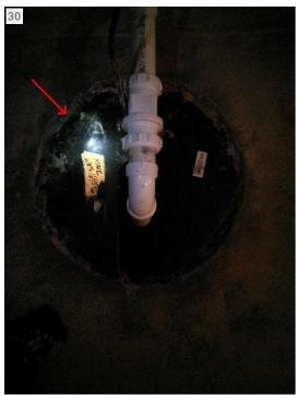
Cement covering lid. Unable to remove to test pump. Have cement chiseled away.
